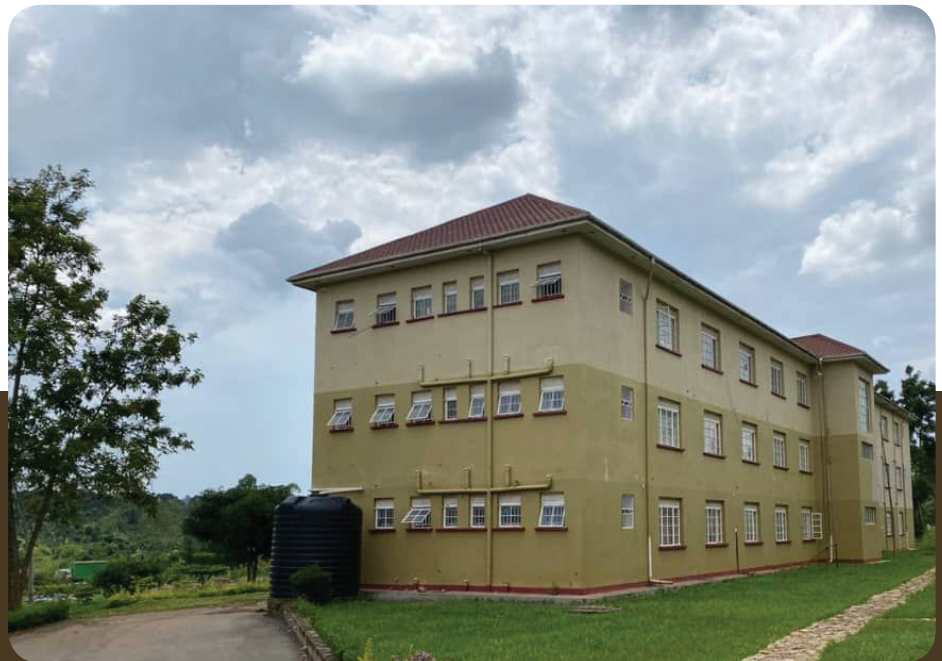
Vision for Africa Intl. high school staff quarters building
